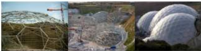
Abbildung 9: Eden Project, Cornwall, GB, Nicholas Grimshaw Architects, Anthony Hunt Associates Ingenieure, Struktur: MERO MembranETFE-Kissen Durchmesser 9 m, Abmessungen: 15 590 m 2 , 100 m x 220 m Höhe 55 (www.anthonyhuntassociates.co.uk).
